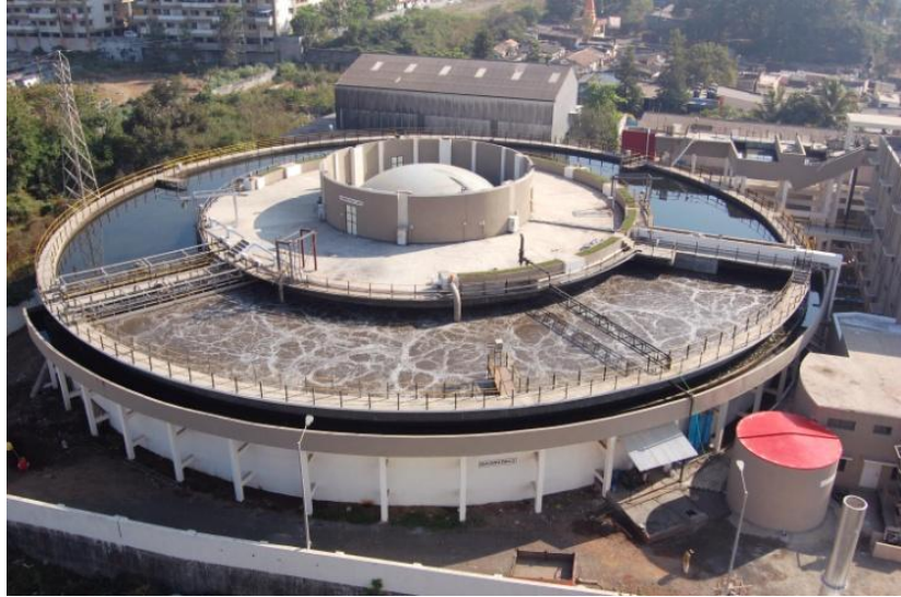
Photograph. 30 MLD capacity STP @ Akurdi, Pune based on Combitreat-ISBR technology
