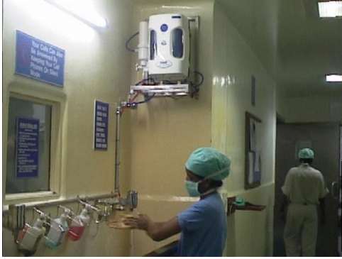
Purioin XL that works on gravity in operation theater (300 LPH)
