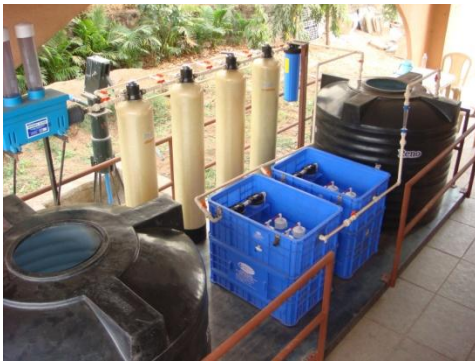
Jal Dhara (5000 LPH /50 KLD) together with iron arsenic /fluoride removal system installed in remote areas of Jharkhand & Bihar
